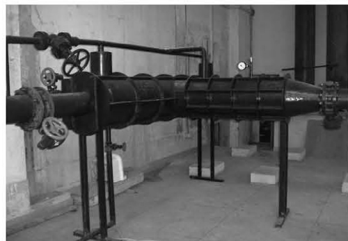
Fig.3 Pressure regulation, exhaust and water control piping
